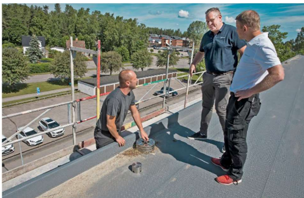
Figur 25. Olivgården Fastighets AB installerar Protan BlueProof tak, Katrineholm.
